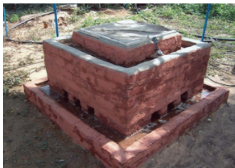
Figure 19. Improved passive cool chamber.
